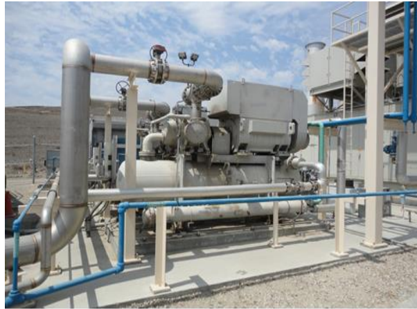
Figure 27. Gas Compressors Arrangement
