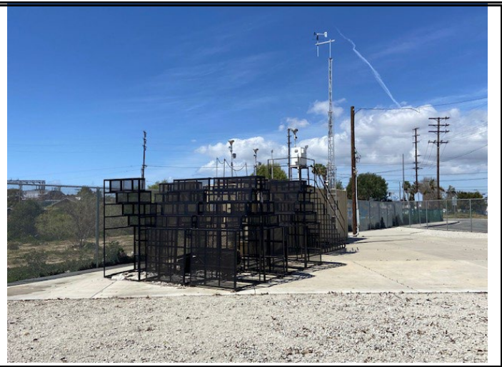
Looking at the probe from the East.
