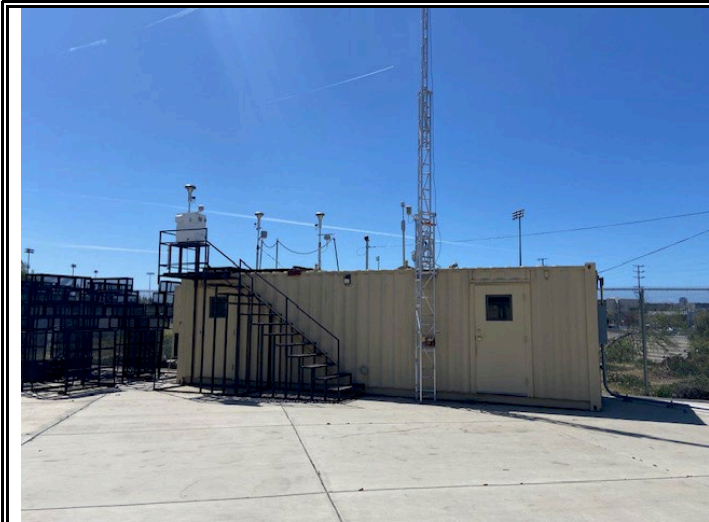
Looking at the probe form the South.
