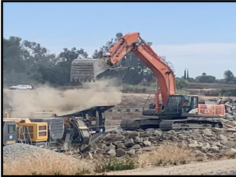
Figure 1-2: Crushing and Grinding Activities at Roadway Project
