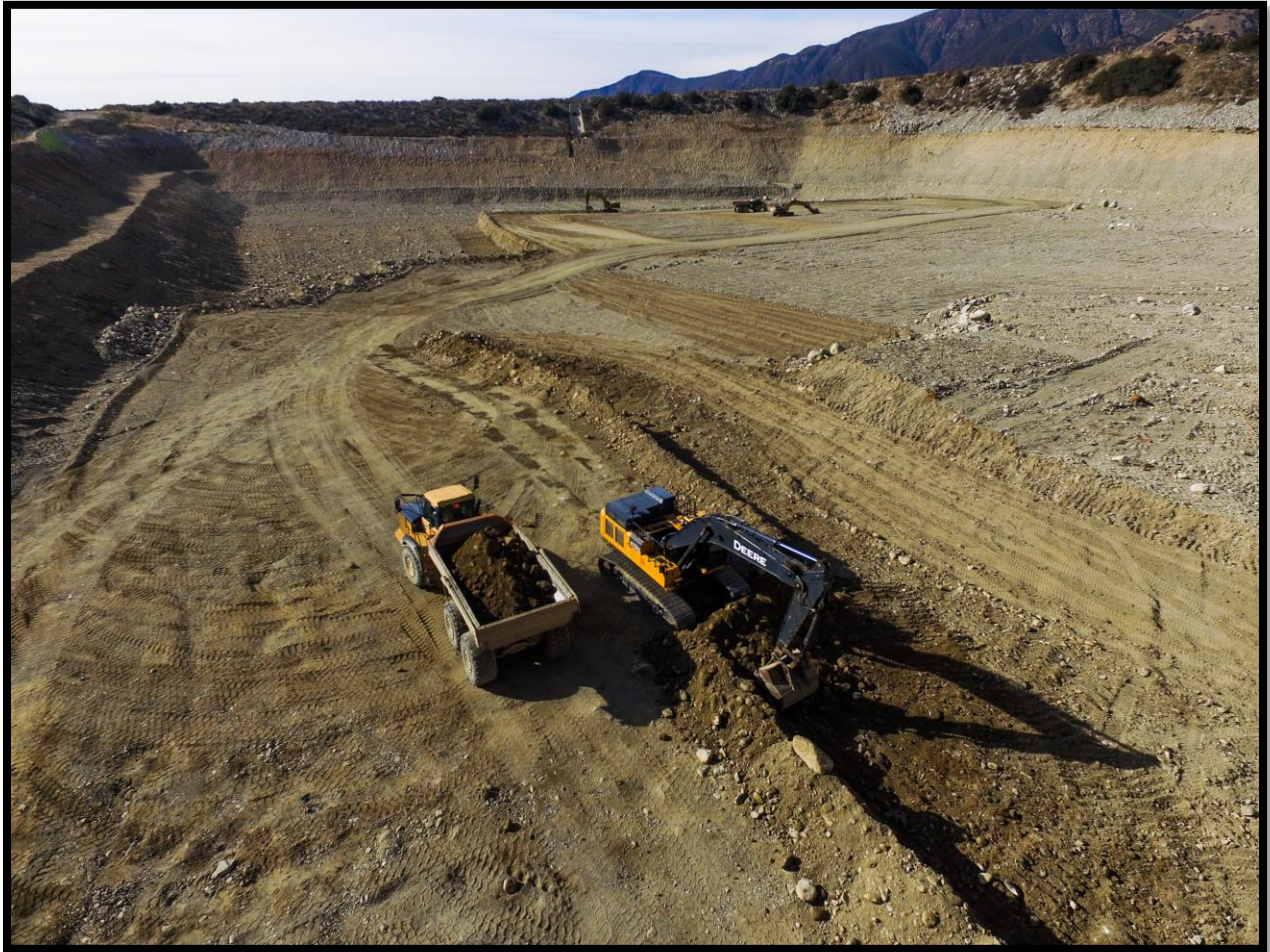
Figure 1-3: Earth-Moving and Excavation Activities
