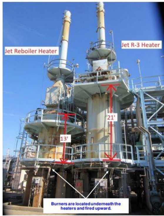
Figure 1-4 Two vertical cylindrical heater configurations.
