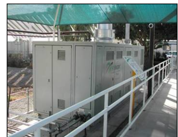
New Reformer Installed
