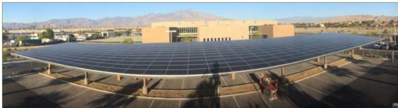
Solar Carport at Sunline Transit Agency
