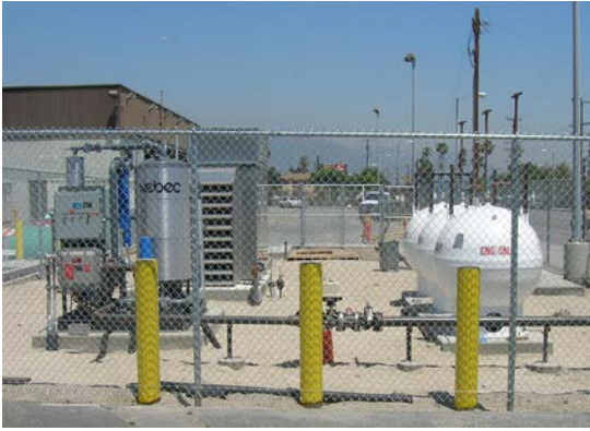
Figure 1: CNG Compressor
