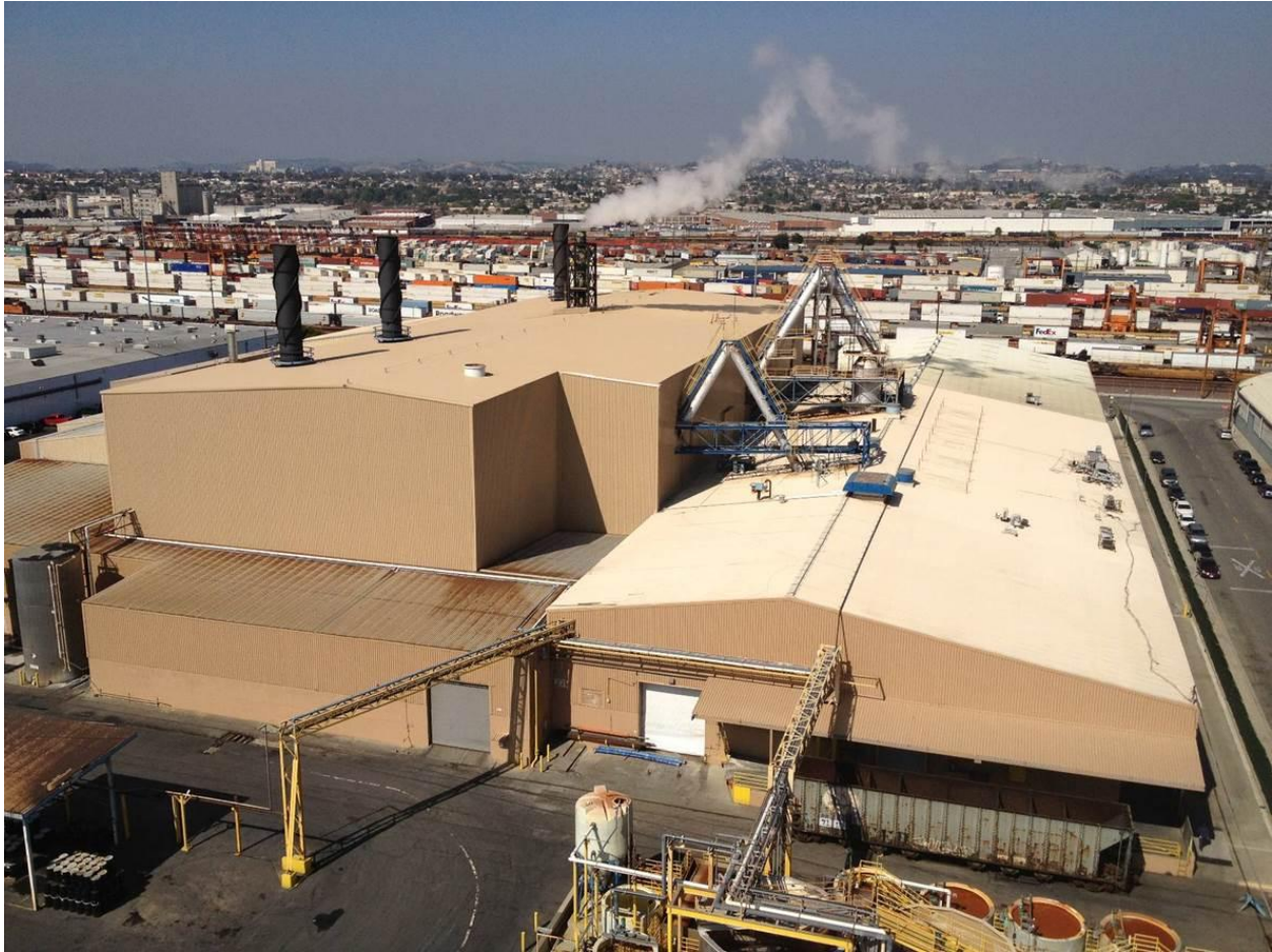
Figure 2-2 Bird's Eye View of Exide
