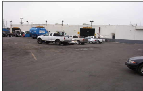
Figure 3: Modified 12 Bay Truck Repair Garage with Gas Detection, Mechanical Ventilation and Alarms
