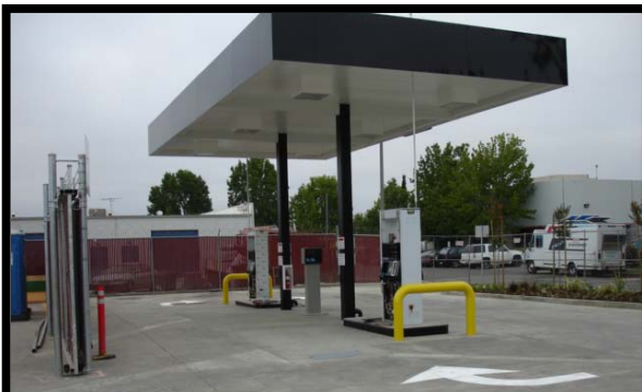
Figure 1: Interior View of Completed Fast-Fill Fueling Island
