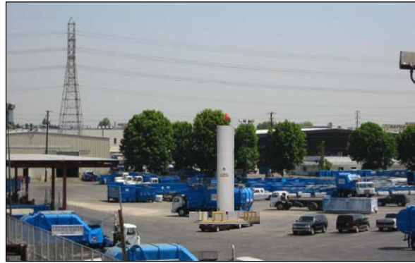
Figure 2: New LNG Facility
