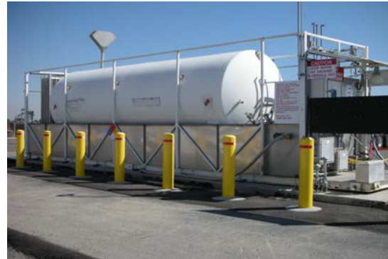
Figure 1: Completed Project Paramount Blvd.
