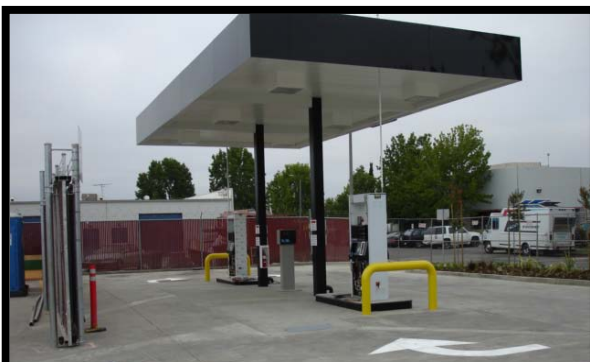
Figure 1: Interior View of Completed Fast-Fill Fueling Island
