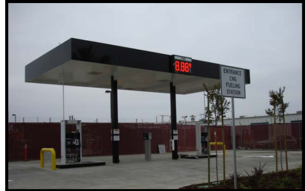
Figure 2: Front View of Fast-Fill Island
