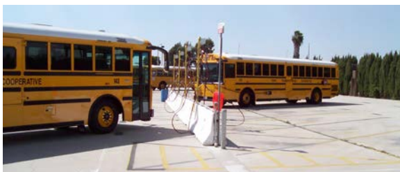
Figure 2: Time-fill Posts Refueling School Buses
