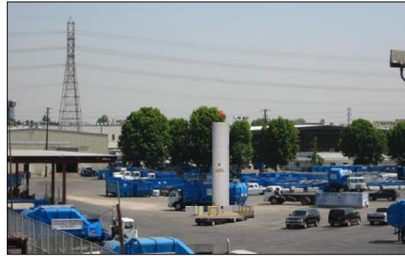
Figure 2: New LNG Facility
