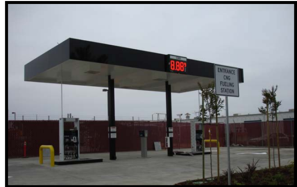
Figure 2: Front View of Fast-Fill Island
