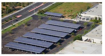
Figure 9: UCR's 4 MWs of Photovoltaic Panels Constructed for Sustainable Integrated Grid Initiative
