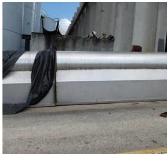
Enclosure around Odorous Operations – The cooker and all processing equipment are housed inside an enclosure. Facility personnel felt an enclosure is crucial to odor containment. One work practice used at the facility is to train operating personnel to close all doors, including access doors and roll-up doors at the entrance to the raw material receiving pits when not in use. This work practice was also considered to be very important to odor containment.
