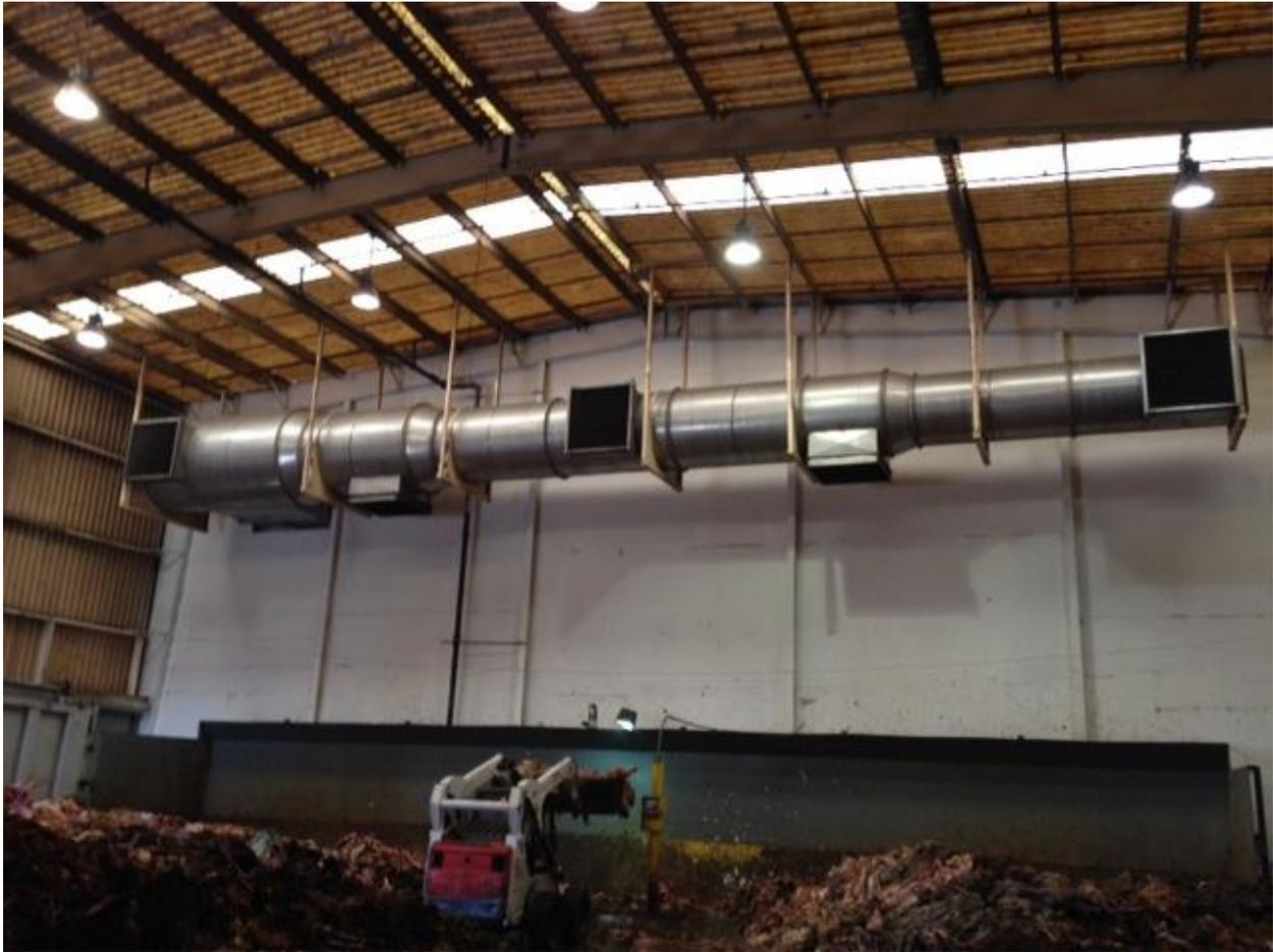
Two rendering facilities have partial enclosures around the receiving area. One consists of a roof with three walls and the fourth wall open. The other has only a roof structure over the receiving pit.
