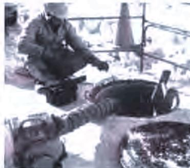
Continuous ventilation and testing are critical in any confined space with a harmful atmosphere.
