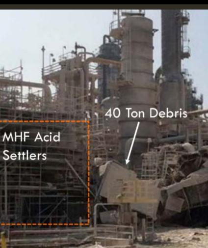
2015 "Near Miss" 40 ton debris lands within 5 feet from MHF tanks at Torrance Refining
