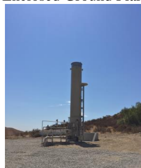
Enclosed Ground Flare
