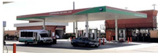
Figure 2: CNG Station after expansion
