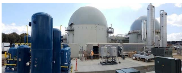
Figure 24: CR&R Anaerobic Digestion of MSW to RNG
