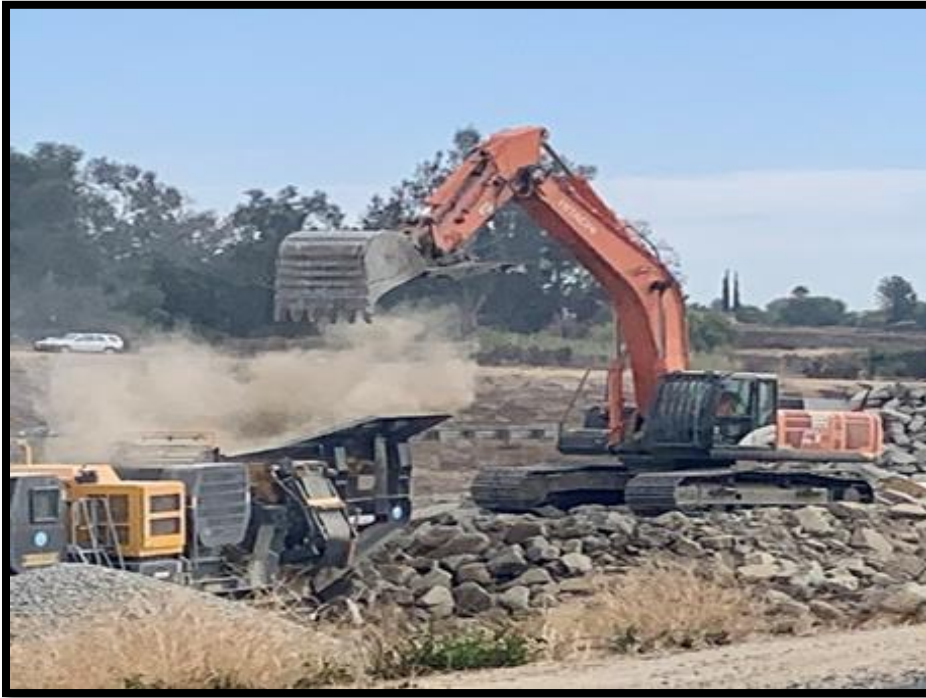
Figure 1-2: Crushing and Grinding Activities at Roadway Project
