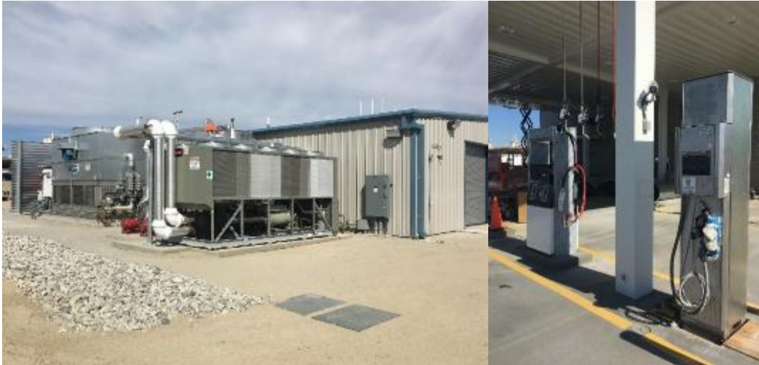
Figure 7: SunLine Transit Agency Onsite Hydrogen Fueling Infrastructure
