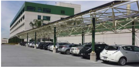
EV charging stations under the solar carport
