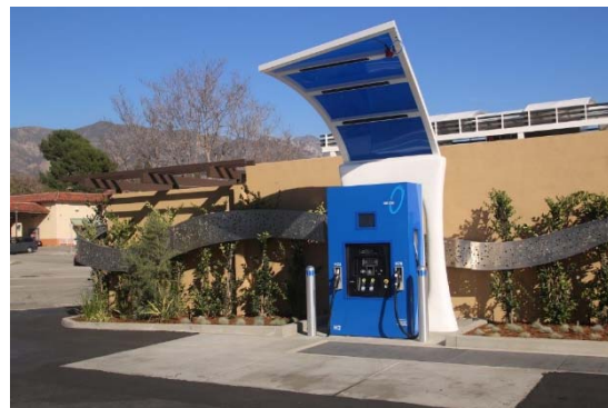
Photo of installed Hydrogen Station at La Canada Flintridge. Source: FirstElement Fuel, Inc.
