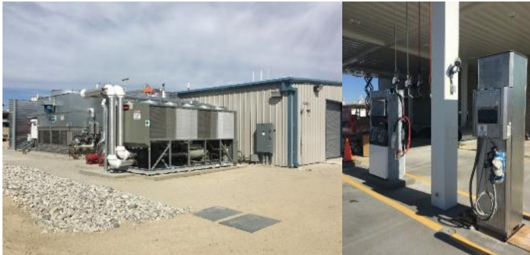
Figure 7: SunLine Transit Agency Onsite Hydrogen Fueling Infrastructure
