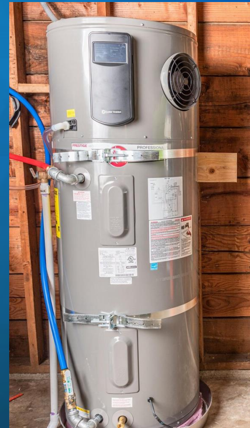
Heat Pump Water Heater
