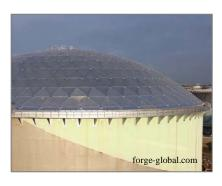
domes on external floating roof tanks storing crude oil can reduce standing losses by 70%-75% 1.
