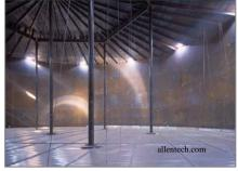
Initially, cable suspended floating roofs were estimated to decrease standing losses by 35%<sup>2</sup>, as based on results from TankESP PRO software. Emissions
