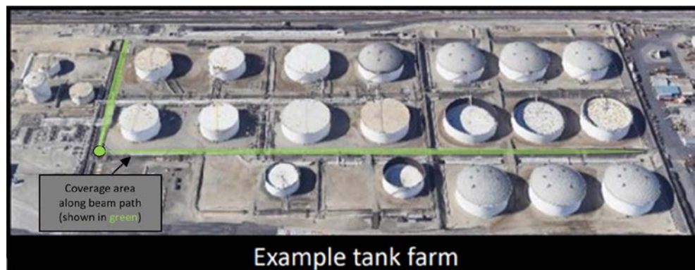
Figure 2.5 – Example of Area Monitored with Open Path Technology
