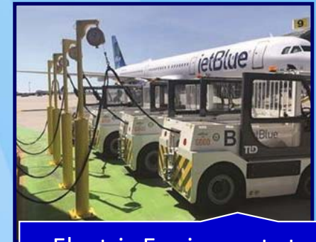
Electric Equipment at Airports
