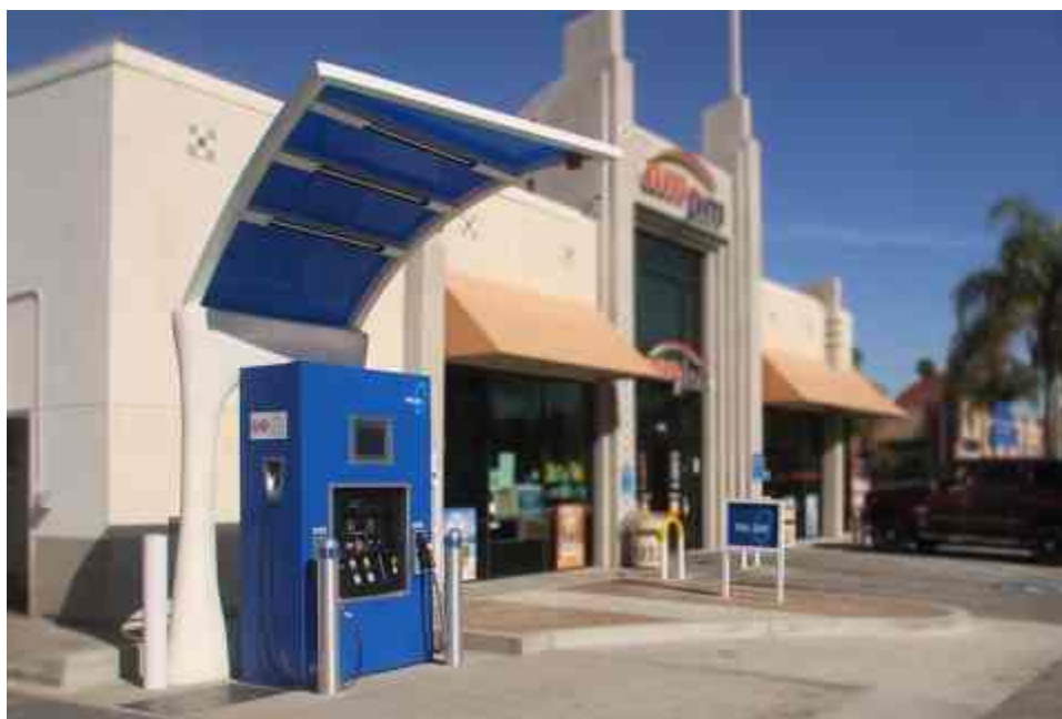
Figure 25: FirstElement Retail Hydrogen Station Co-located at ARCO Gas Station in Long Beach
