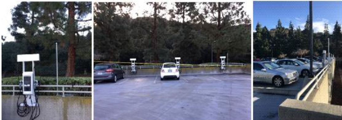
Figure 32: Installations in Progress
