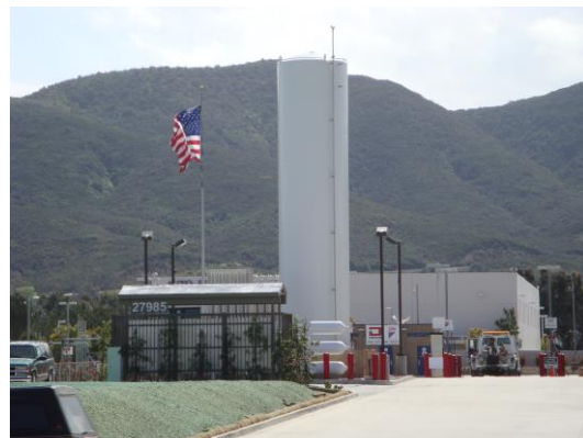
Figure 1: CNG Station in Temecula
