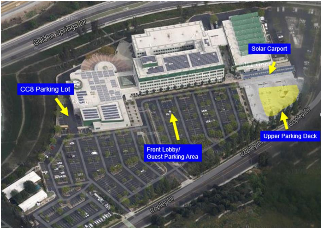
Figure 31: Areas of EV Charger Installations at SCAQMD Headquarters
