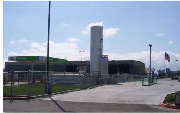
Figure 1: Upgraded Agua Mansa L/CNG Station
