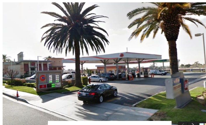
Figure 19: Ontario CNG Station
