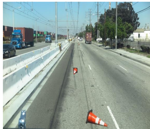
Figure 17: eHighway Infrastructure on Alameda Street
