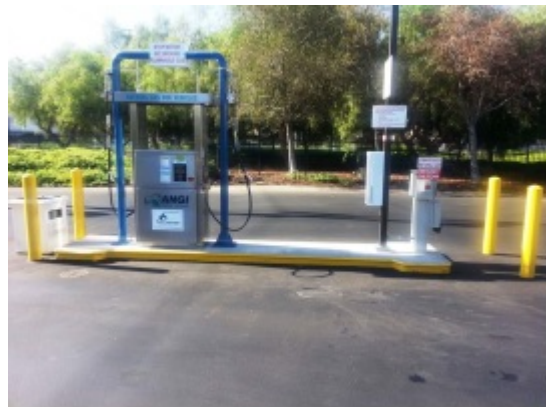
Figure 1: New Dual-Hose Fast-Fill Dispenser
