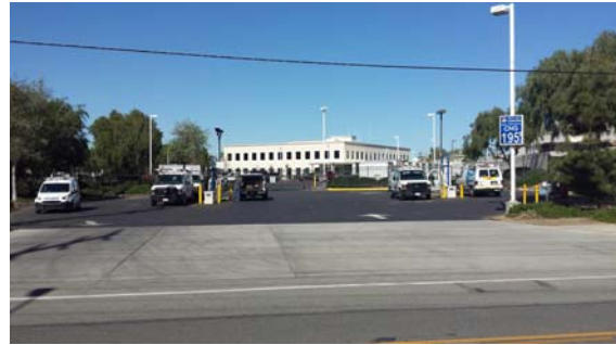
Figure 3: Station after Upgrade
