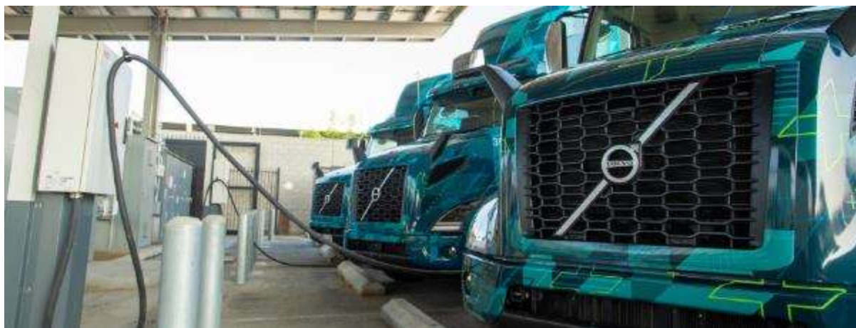
Figure 24: Three Volvo VNR Trucks Charging at DHE in Ontario
