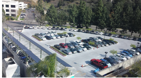
Level 2 Chargers on Upper Parking Structure
