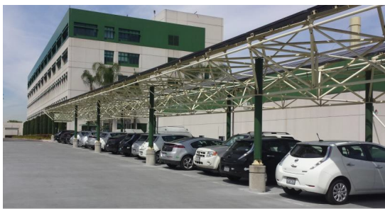
Level 2 Chargers Under Solar Carport
