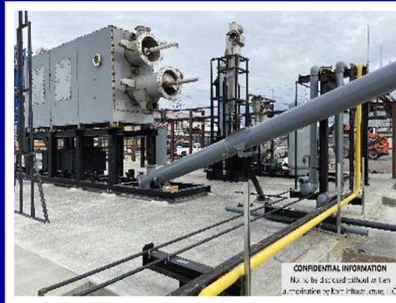
Pyrolyzer, Feed Conveyor, Char Conveyor, Gas and Water Piping efforts
