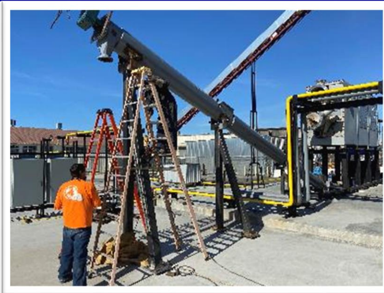
Pyrolyzer, Feed Conveyor, Char Conveyor, Gas and Water Piping efforts
