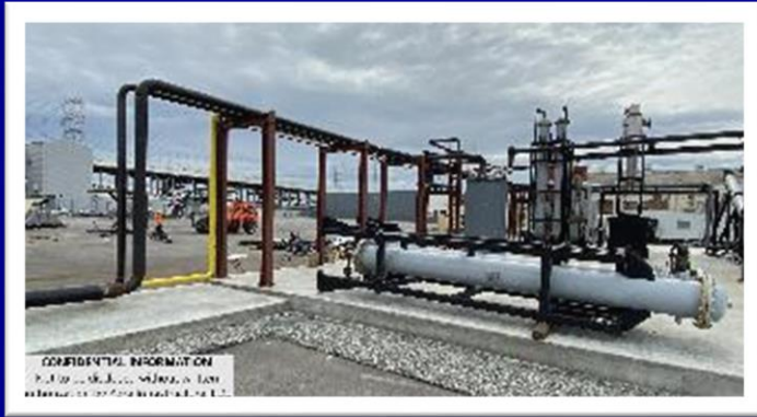
Piping efforts, North view
