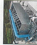
Industrial Example of a Finned Tube Heat Exchanger
