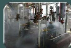
Water Spray for Pump Deluge
