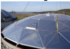
Current requirement: Doming for all tanks storing liquid with true vapor pressure of  $\geq 3$  psia, including crude oil tanks, crude oil tanks exempt
