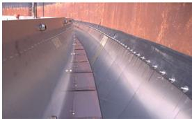
Current requirement: Secondary seals not required for internal floating roof tanks; gap allowances for primary seals up to 30% or 60% of tank circumference, depending on gap size
