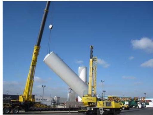
Figure 1: LNG Tank Installation
