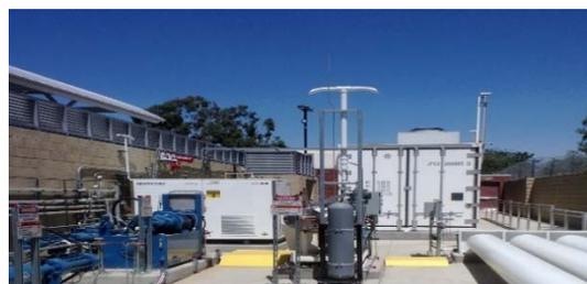
Figure 1: CSULA's H<sub>2</sub> Station interior (from left to right): high pressure compressors, H<sub>2</sub> chiller, 350 bar compressor, electrolyzer, 350 bar storage banks, visitor gallery
