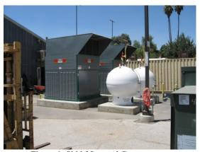
Figure 1: Skid-Mounted Compressors and CNG Storage Spheres
