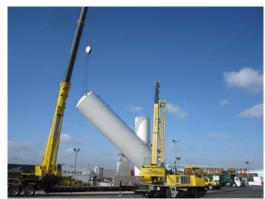
Figure 1: LNG Tank Installation
