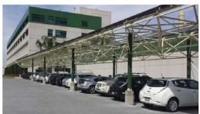
Figure 2: SCAQMD solar carport featuring upgraded EVSE
