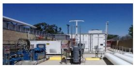
Figure 1: CSULA's H<sub>2</sub> Station interior (from left to right): high pressure compressors, H<sub>2</sub> chiller, 350 bar compressor, electrolyzer, 350 bar storage banks, visitor gallery
