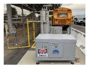
Figure 1: BRC FuelMaker FMQ-8-36
