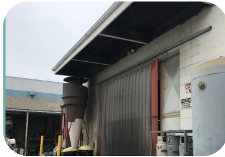
Cross-Draft Minimization Using Overlapping Strip Curtains
