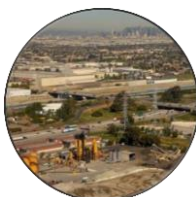
General Industrial Facilities
