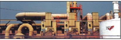
Collection of secondary lead oxide emissions using four FEF SERIES units.
