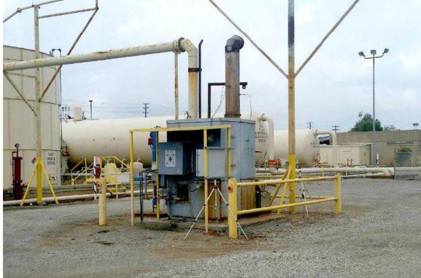
**Figure 2-12. Existing Thermal Oxidizer at the 700 Block**
