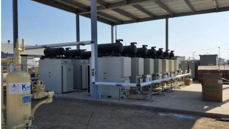
**Figure 2-17. Breitburn's Microturbines.**
