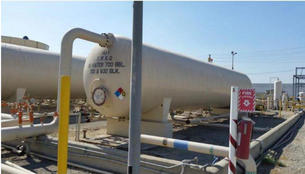
**Figure 2-5. Free Water Knock Out Vessel at the 700 Block Main Facility.**
