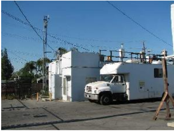
Looking at the probe from the North.
