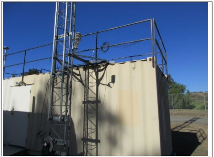
Looking at the probe from the East.
