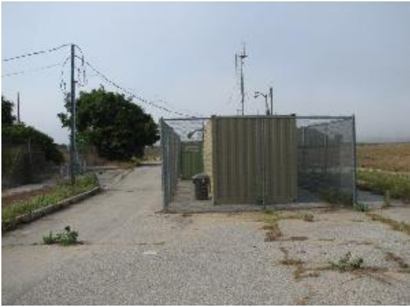
Looking at the probe from the North.
