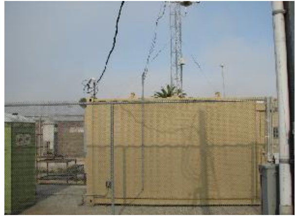
Looking at the probe from the East.
