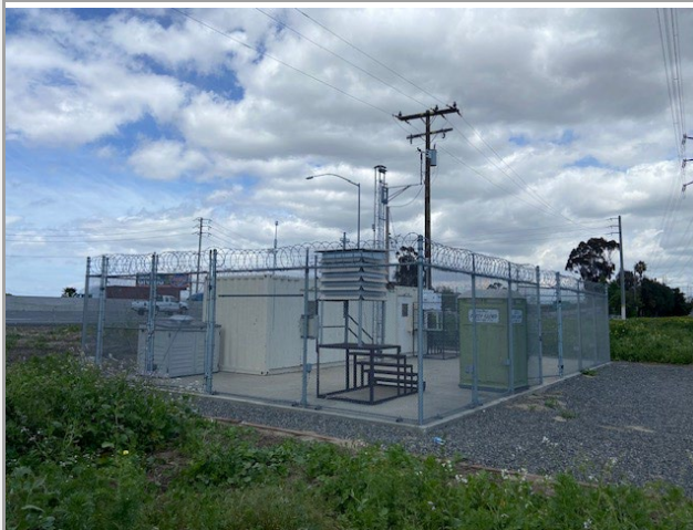
Looking at the probe from the South.
