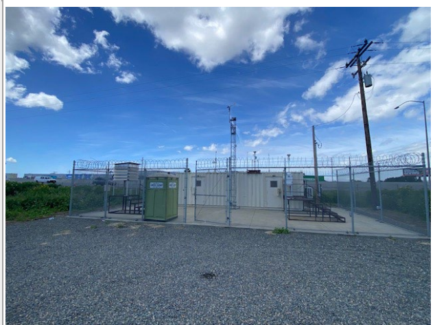
Looking at the probe from the East.
