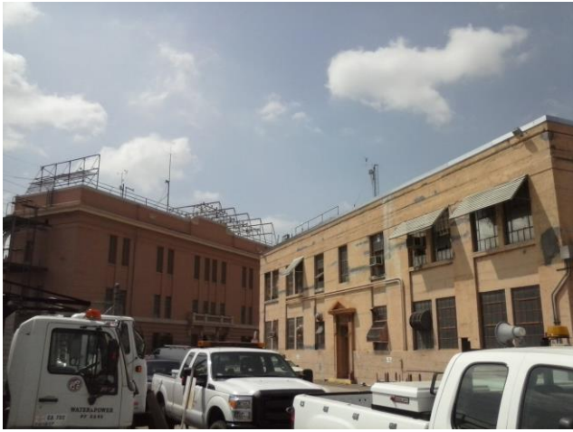
Looking at the probe from the North.
