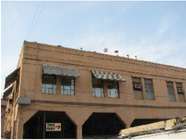
Looking at the probe from the North.
