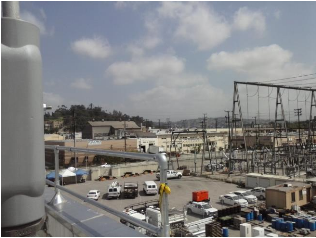
Looking North from the probe.
