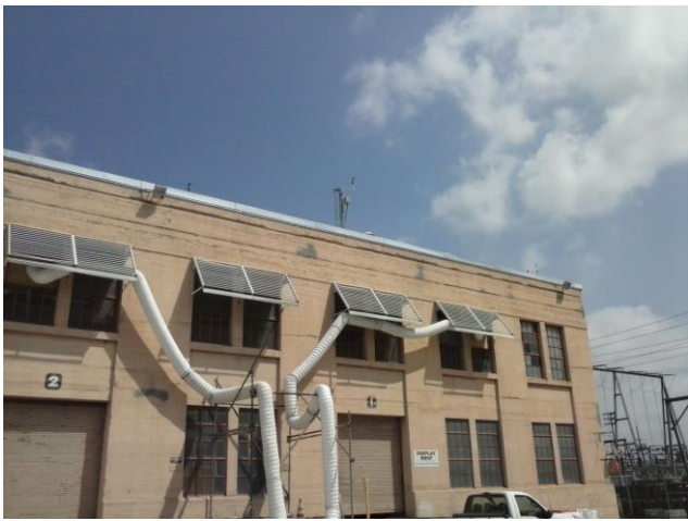
Looking at the probe from the South.
