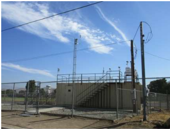
Looking at the probe from the South.
