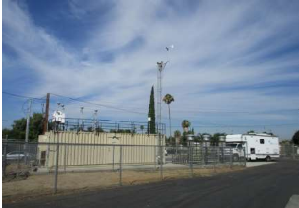
Looking at the probe from the East.
