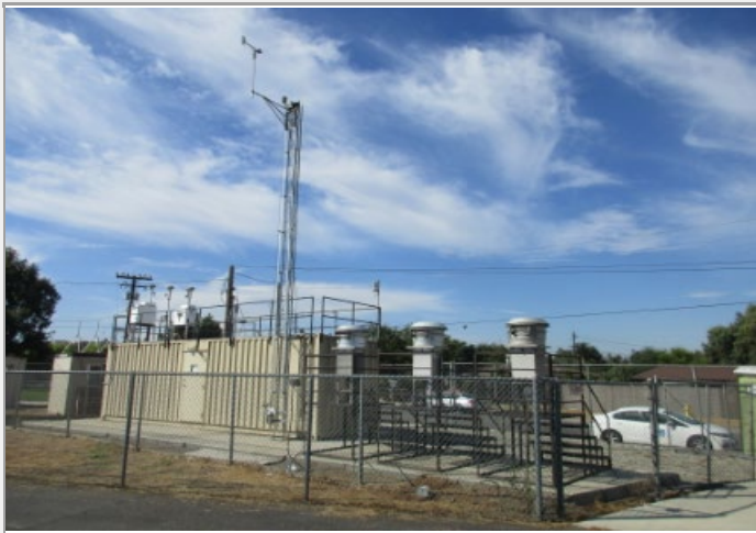
Looking at the probe from the North.
