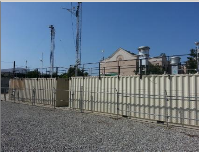
Looking at the probe from the South.
