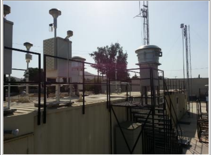
Looking at the probe from the East.
