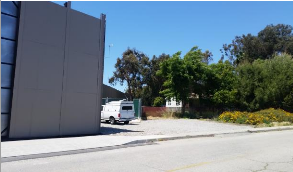
Looking at the probe from the South.
