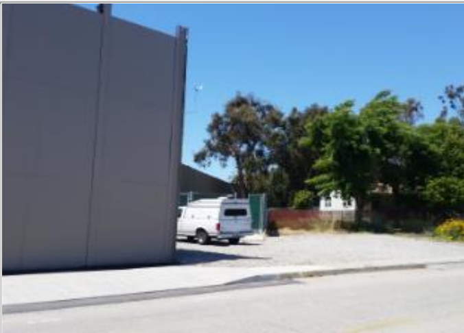
Looking at the probe from the South.
