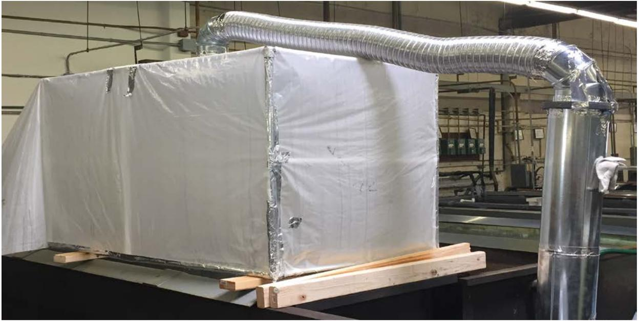
Figure 1 - Photograph of Temporary Ventilation System with Sampling Location.
