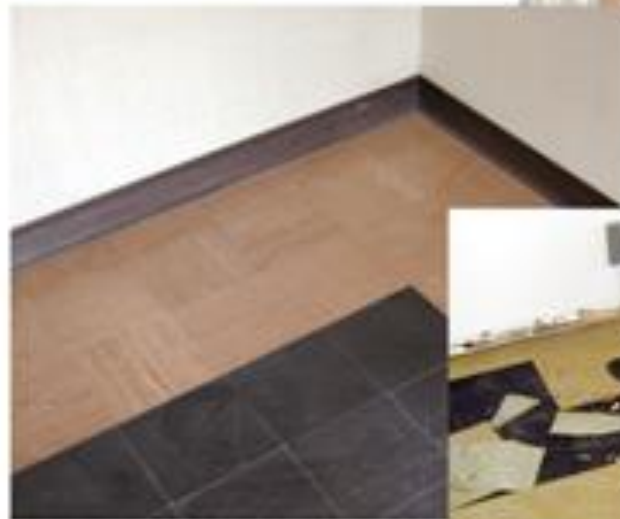
9" VINYL ASBESTOS TILE (LEFT) & BLACK ASBESTOS MASTIC (BELOW) EXPOSED DURING CARPET REMOVAL
