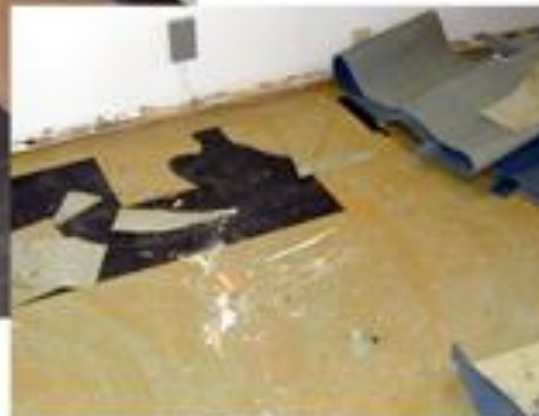
9" VINYL ASBESTOS TILE (LEFT) & BLACK ASBESTOS MASTIC (BELOW) EXPOSED DURING CARPET REMOVAL
