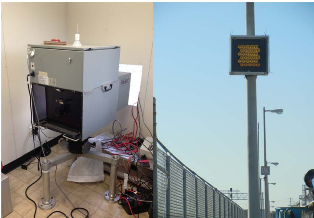
Figure 6.1: Photograph of the IMACC FTIR at the Carson FML (left) and retroreflector mounted at the light post inside the Tesoro refinery (right).
